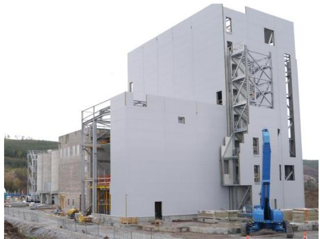
The Helius CoRD project near Rothes on Speyside is a new facility to provide energy by incineration of timber and spent barley 'draff' produced as a residue of the whisky process. Melia Smith & Jones were appointed as the Owner's Civil Engineer and oversaw the foundation works on site.
