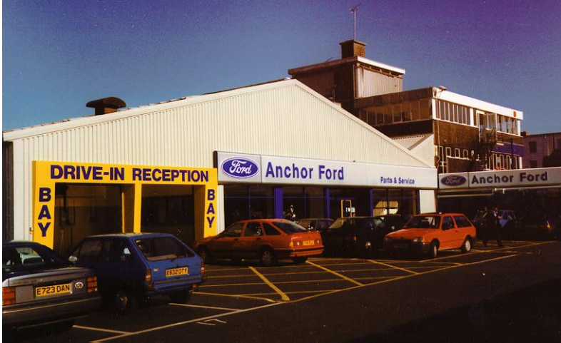
Anchor Ford - a refurbishment project in Reading.
