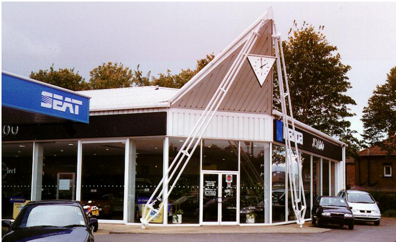
JCT - a new build site on vibro compacted ground in Leeds
