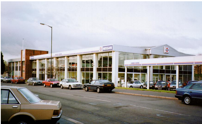
Nissan - a refurbishment and extension of industrial buildings in Bristol.
