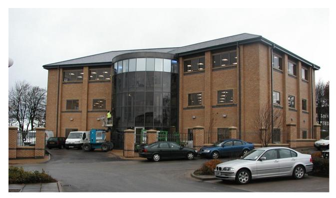
The project involved construction of a new 3-storey office building within an existing business park in Harrogate. The requirement was for clear open space with raised computer floors. The steel framed superstructure utilised cellular beams, composite with the floors, to achieve the clear spans and allow future installation of air conditioning ductwork.
