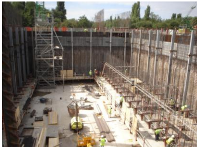
Bunker slipform set-up - Lakeside EfW
